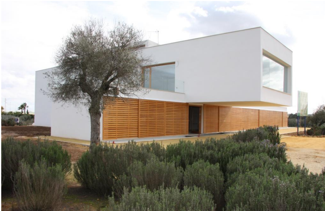
Image 4. Main building at the CENTA facilities.
